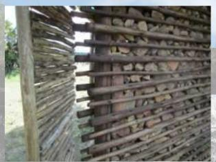
A lattice wall, filled with rock or another medium kept moist during the hot hours of the day, acts as an amazing natural air conditioner. Cover it with a canvas screen against drafts at night, and it becomes an equally efficient heater radiating the sun's stored energy. To top it all, it should only cost you a fraction of a conventional wall! Metal piping in the boma floor to heat water and a donkey boiler in the braai chimney are some of the other original ideas that our owners came up with.
